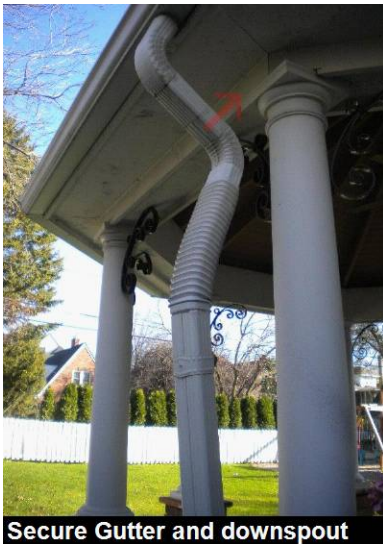
Secure Gutter and downspout
