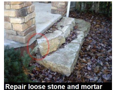
Missing mortar
