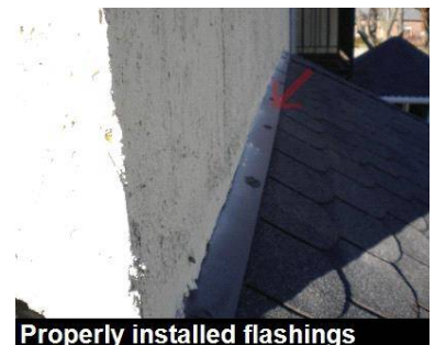
Properly installed flashings
