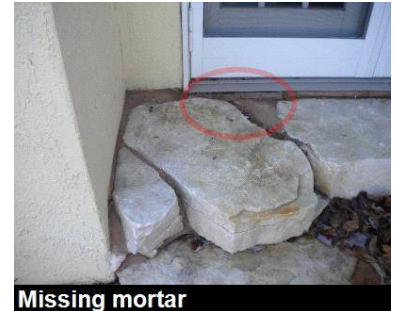
Repair missing mortar
