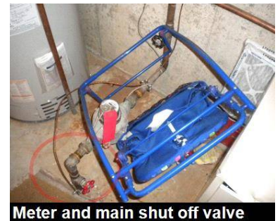
Meter and main shut off valve
