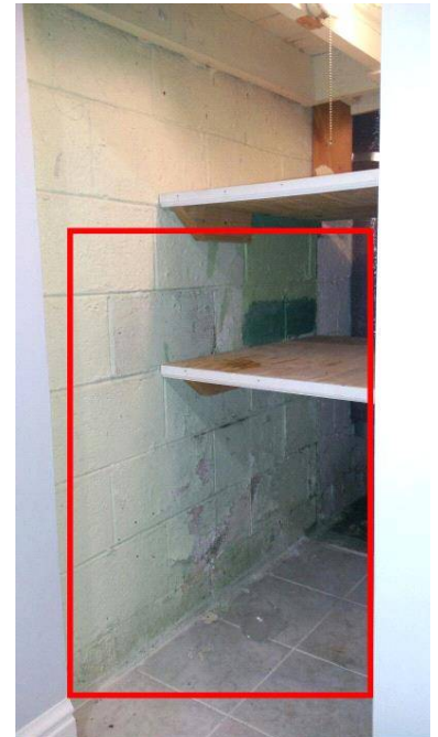
Moisture damage is noted
