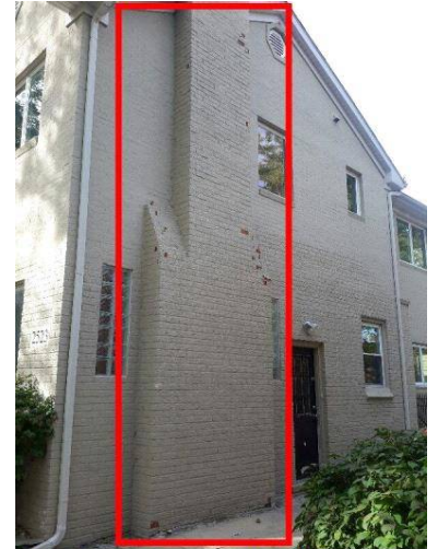
Maintain damaged brick facing
