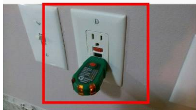
GFI Outlet failed trip test
