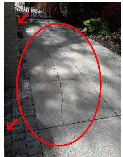
Noted Cracks are typical / Seal Drive Wall
