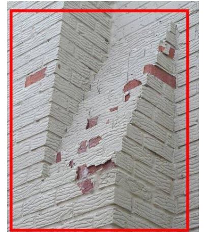
Maintain damaged brick facing
