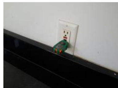
Missing cover plate / Trim ring
