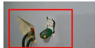
Missing cover plate / Trim ring
