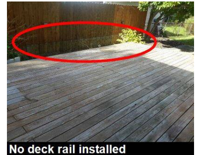
No deck rail installed
