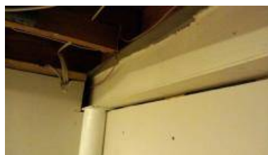
High moisture content noted in walls
